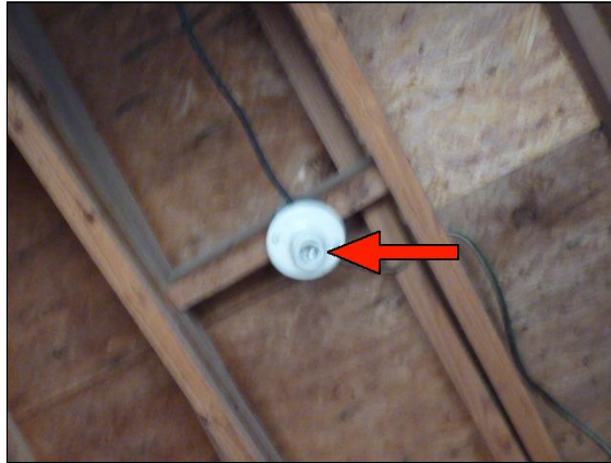
Attached storage shed interior ceiling fixture
